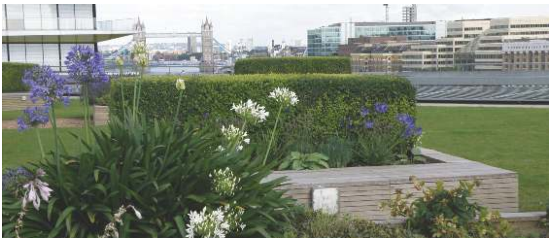
Angel Lane, an intensive green roof
