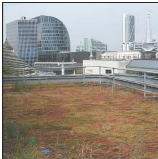
1 Wood Street; an extensive green roof
